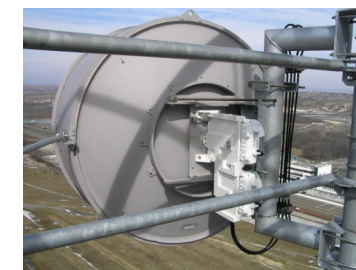
(3+1) system under construction (2 ODUs installed)
