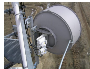
(3+1) system under construction (2 ODUs installed)
